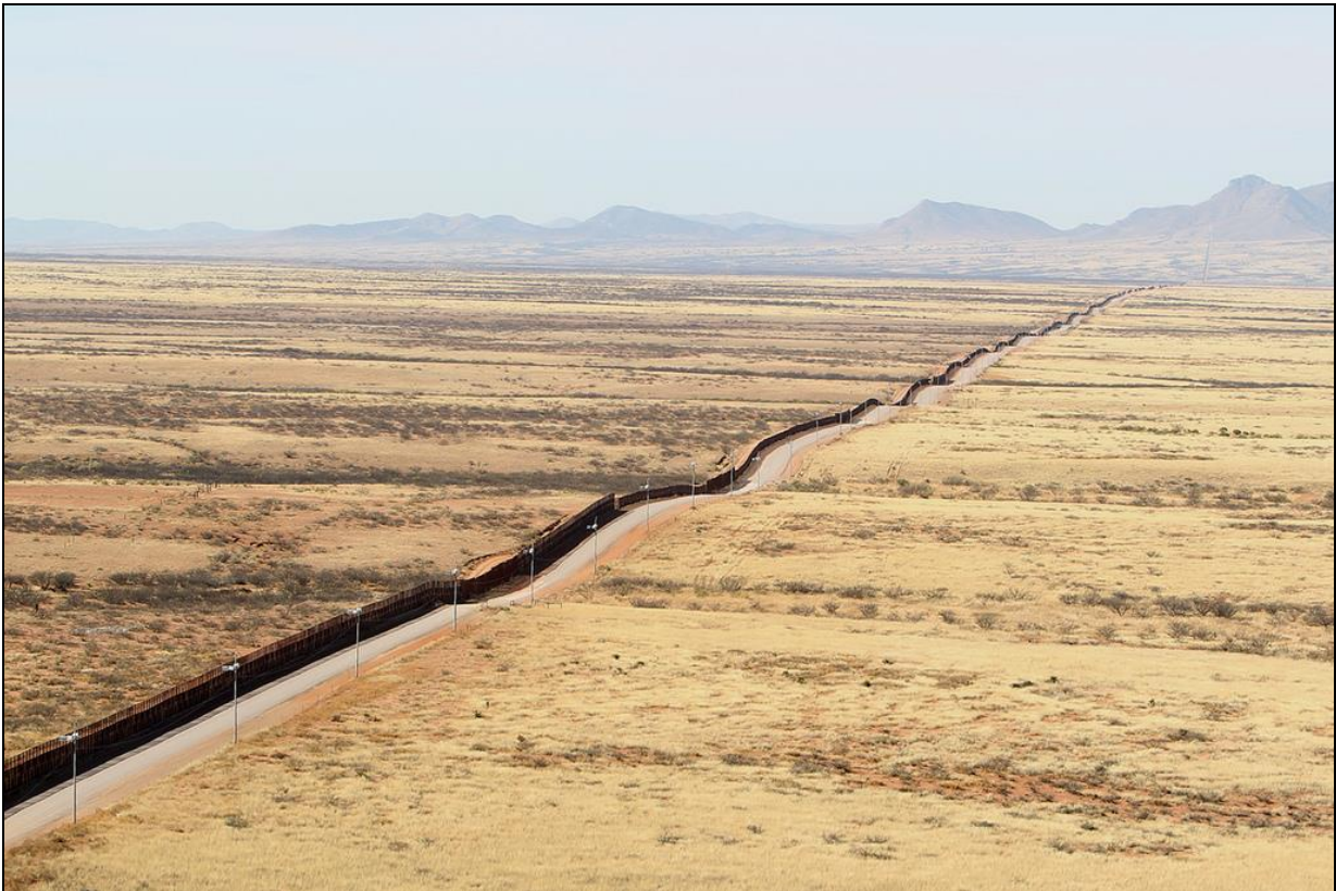
Border fence along the Arizona-Sonora boundary Photo courtesy U.S. Customs and Border Protection
