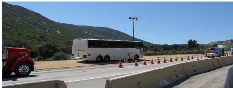
Figure A.26. I-8 checkpoint secondary screening area. Secondary screening for busses is on a dirt shoulder near a steep decline. Secondary screening for passenger vehicles is to the right of the cones in the photo. (Source: UA)
